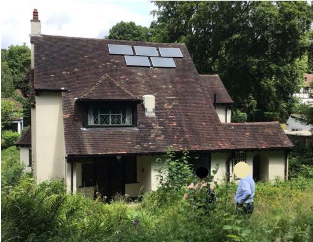
Figure 3: Rear of existing dwelling
